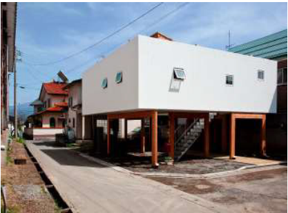
HOUSE BB | 2009 Private House | Nagano, Japan
