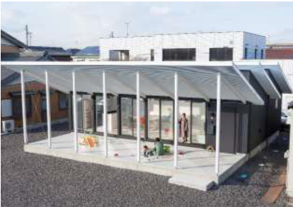
Saw-Tooth Roof in Ichinomiya | 2017 Private House | Aichi, Japan
